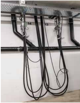
The supply hoses for the coolant and compressed air
