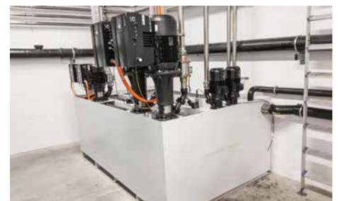
Part of the tank system in the cellar of the new building
