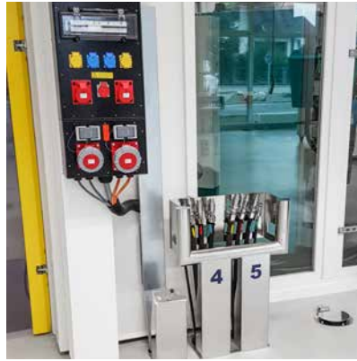
GIFAS power boxes and coolant pumps, as well as compressed air connection and drain for coolant
