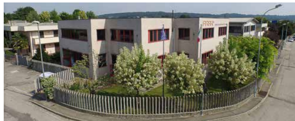
AFAR company headquarters in Sesto Calende, Lombardy, Italy
